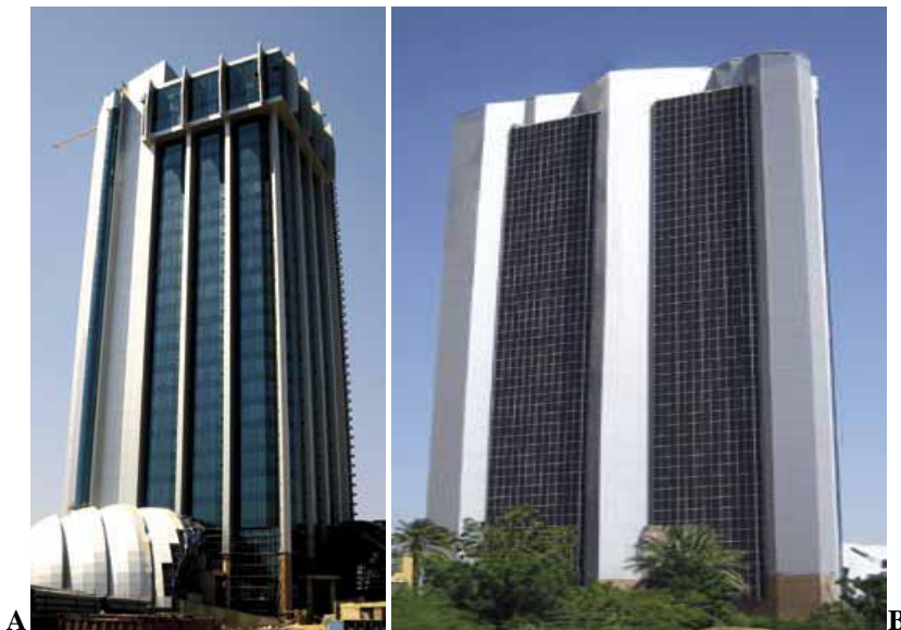
Figure 14: A shows see through thin film type Figure 13: B shows opaque thin film type
