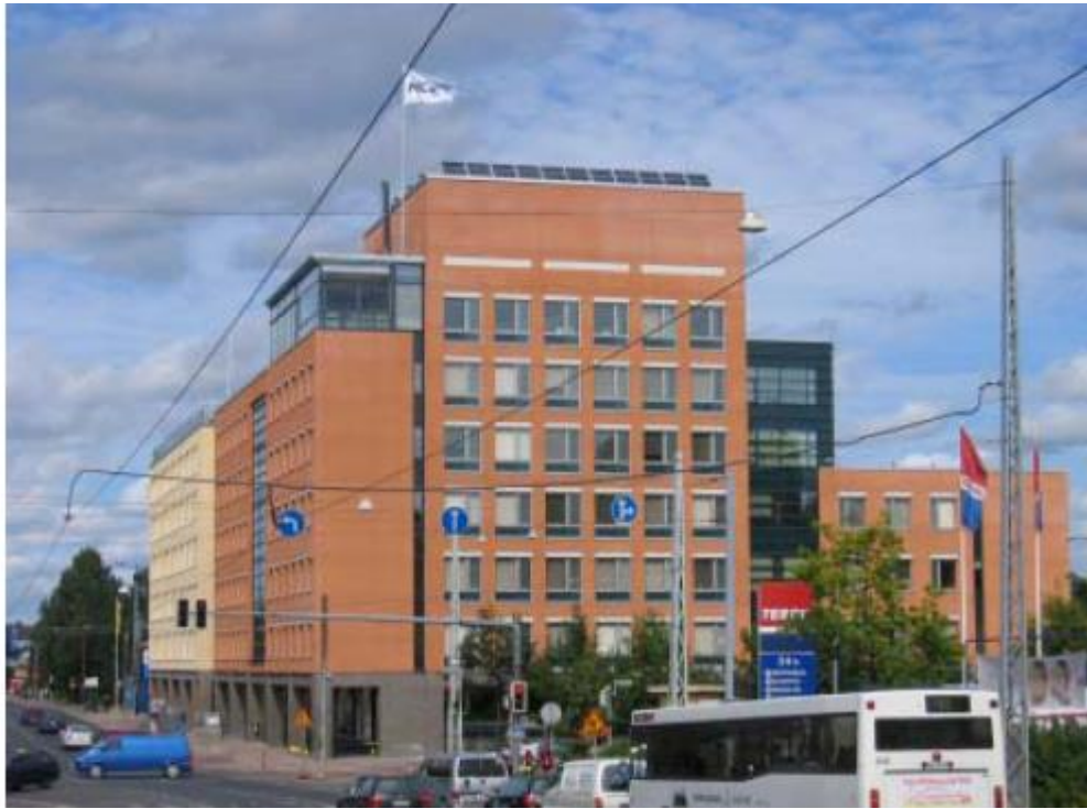
Figure 14: NCC head office.( Amogpai, A ,2011)
