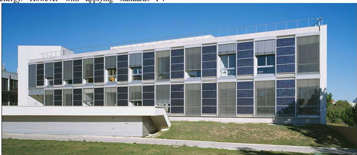
Figure6 : PV integrated into the opaque parts of the façade Credit: http://csc.esbensen.dk/ .
