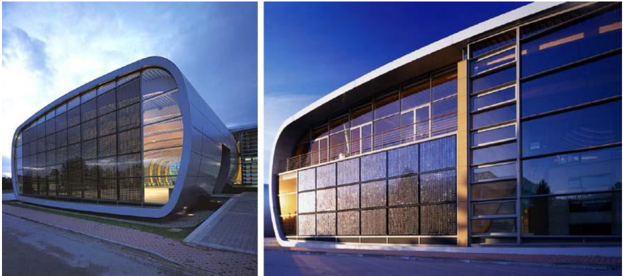
Figure 7: Tobias Grau Production Building in Germany has PV integrated into its south glazed facade Credit: http://csc.esbensen .
