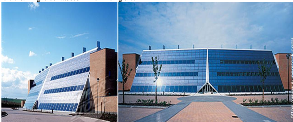
See figure 9: PV integrated inclined wall of Daxford Solar Office Credit: superstock.com/
