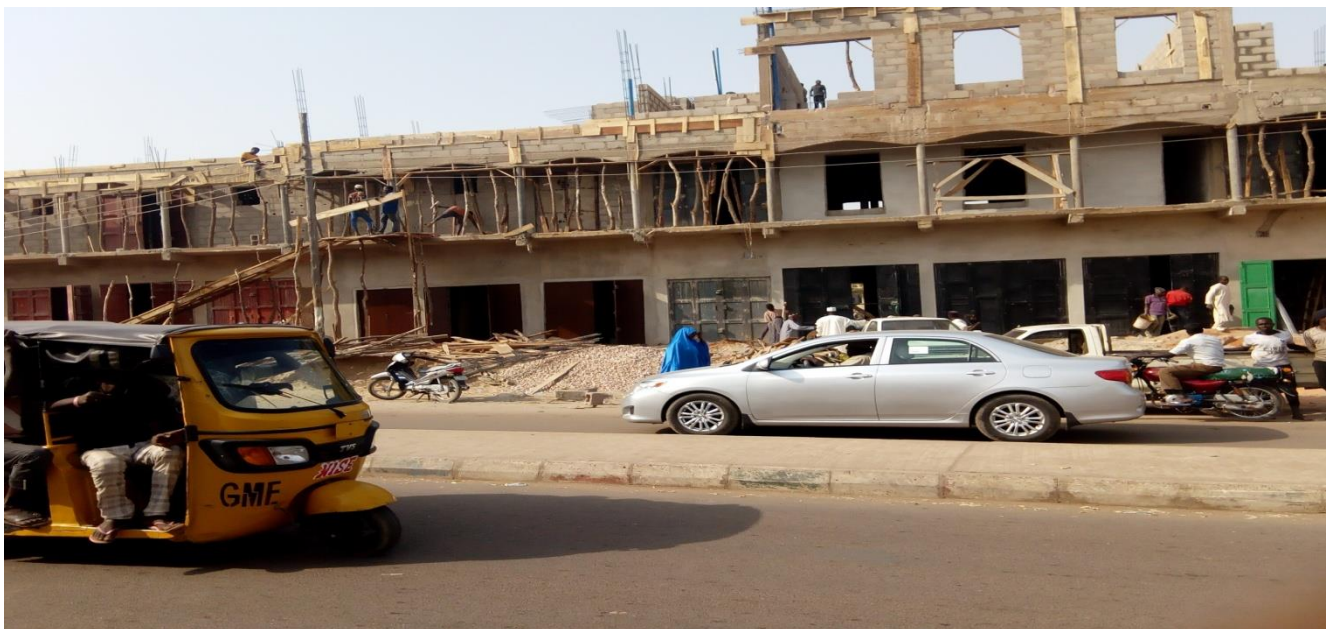
Picture 5: Building Construction in progress (Gombe Metropolis).
