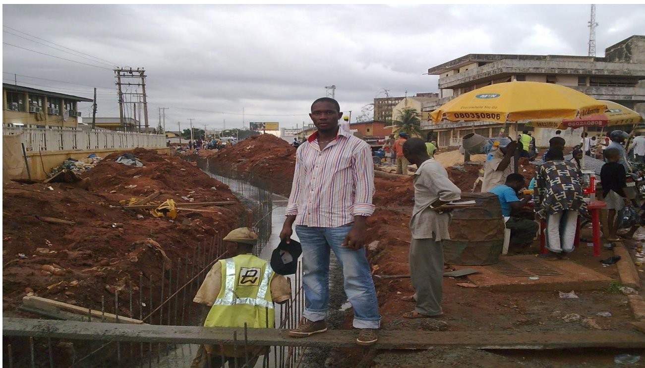
Picture 2: Construction workers casting drainage base.
