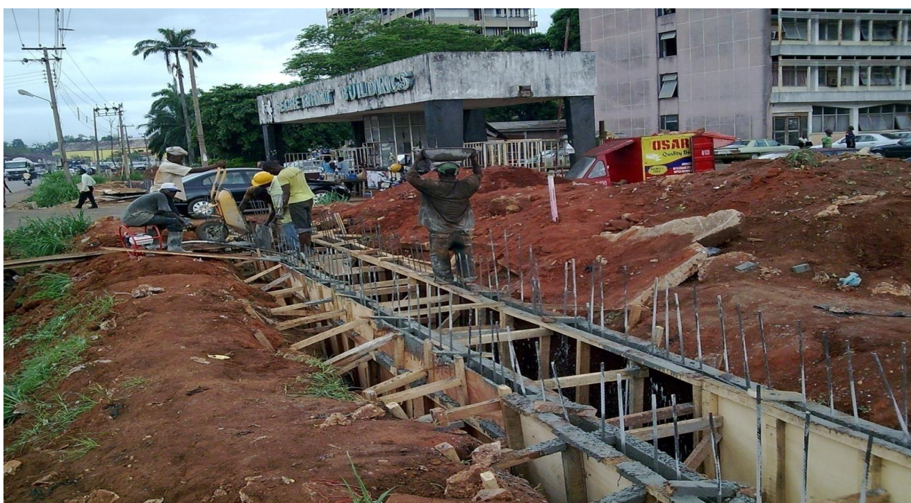
Picture 3: Construction workers casting drainage walls.
