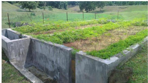
Fig. 4 Outlet of Bioretention
