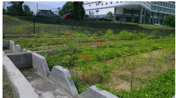
Fig. 3 Inlet of Bioretention
