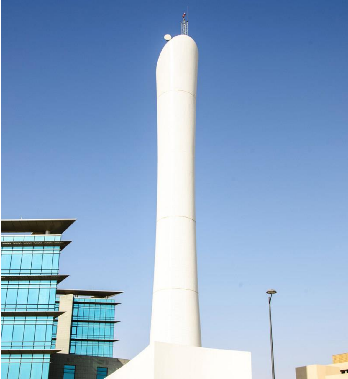
Figure 2 GSM Greenfield Camouflaged/Monopole Model (Al-Babtain Power & Telecom, 2021)
